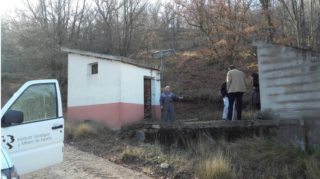
Manantial 1 "Masegal". Vista exterior
