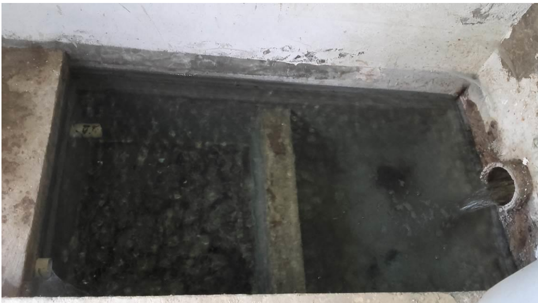
Manantial 1 "Masegal". Vista interior
